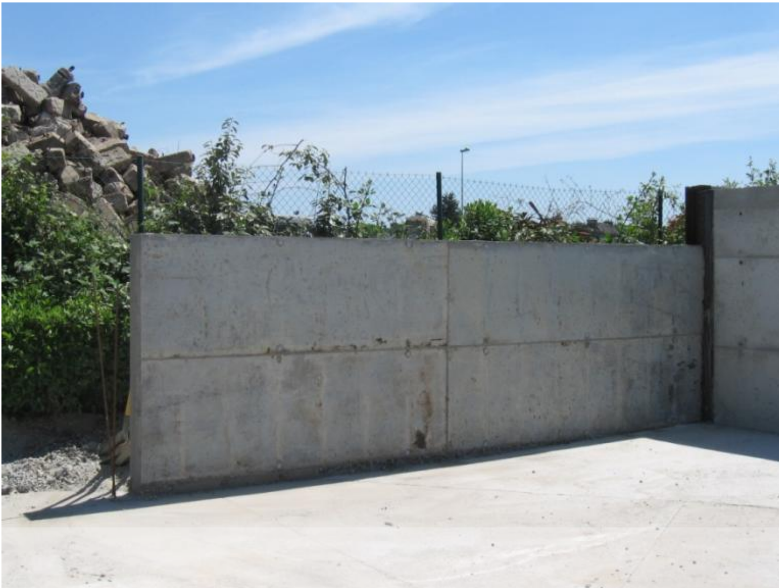
Promptis® - Fast Form Removal Demoulding after 4h
