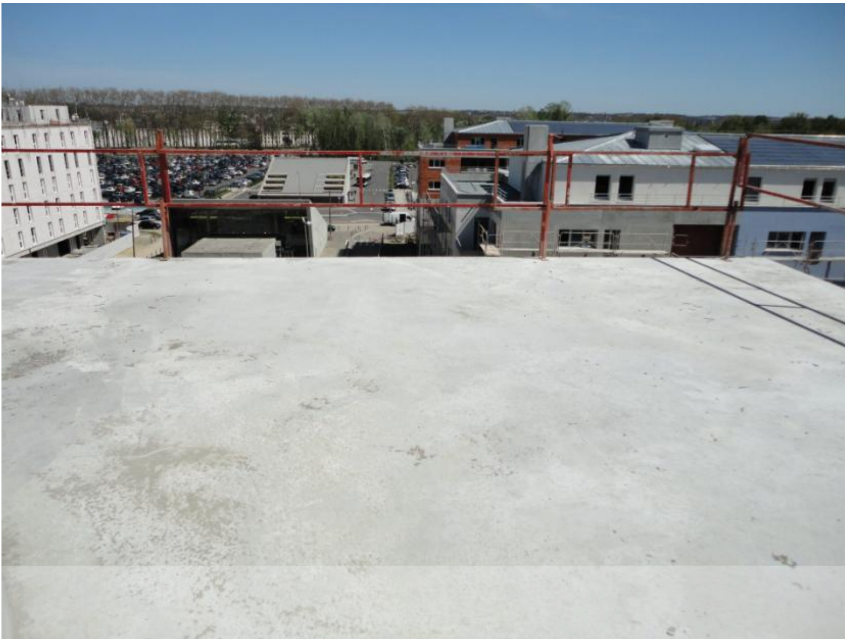
Finishing concrete of Promptis® after 4 days.
