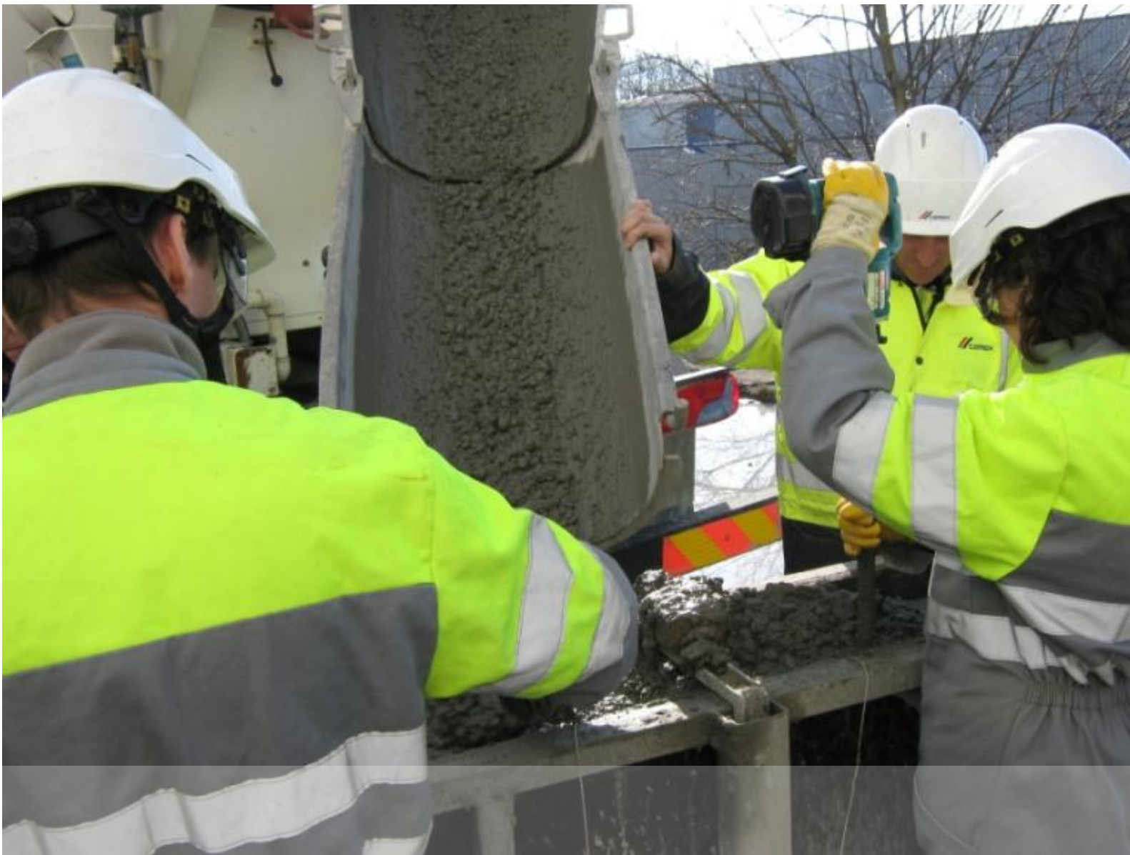
Casting and placing S3 consistency concrete after 1h of workability retention
